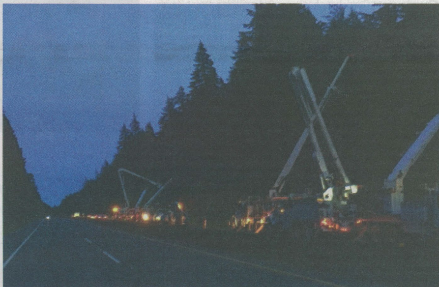
Safety comes first with a barrier placed between traffic and crew during a night time repair of power lines bordering a highway
